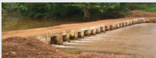
Bablaie Mata Bridge, Juvi Nala Bhamragad
